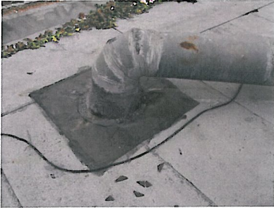
7. ACM black mastic associated with roof penetrations, totaling about 50 ft 2 [Sample I.D. RFMAS-05-01, -02, -03, containing 4% Chrysotile asbestos (CH)].
