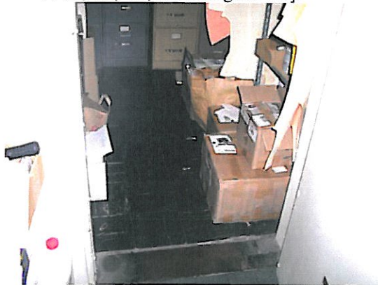
16. ACM 9” x 9” black vinyl floor tiles with tan streaks and associated black mastic (typically concealed beneath carpet), totaling about 2,400 ft 2 [Sample I.D. FLVCT-23-01, -02, -03, containing >1% CH in the tiles, 3% CH in the mastic].
