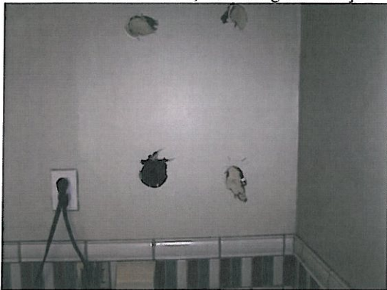
15. ACM black mirror mastic on a wall (mirror absent), totaling about 1 ft 2 in the Men’s Restroom [Sample I.D. MASTIC-19-01, containing 10% CH].
